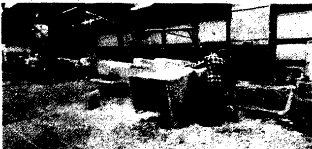
Workers applying fiberglass to another shower unit. (See finished product above.)
